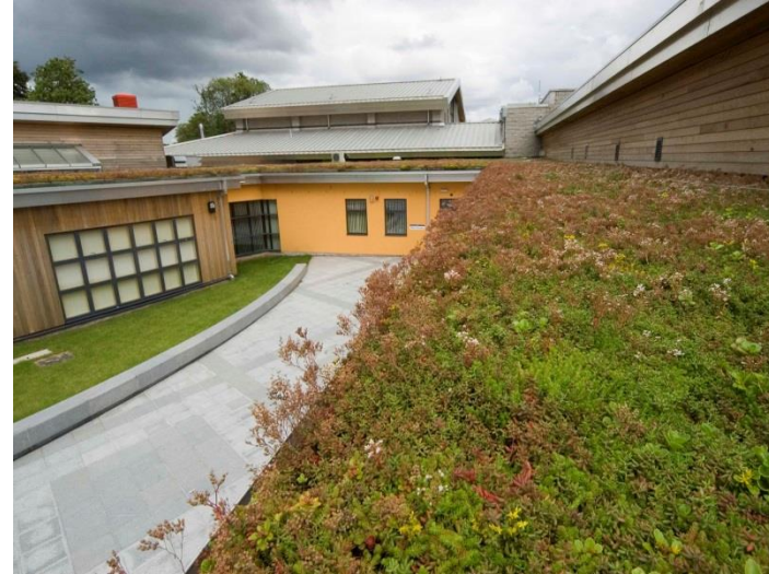
Green roof, Kinnaird Primary School
