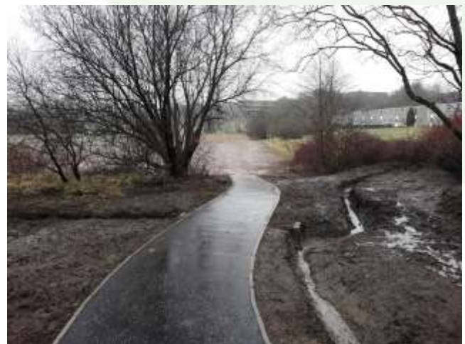
After the new path and drainage was installed
